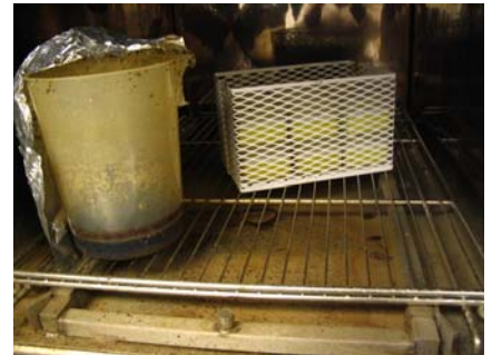
LIQUID RUN ON SOLIDS CYCLE— (NOTE BOIL-OVER IN CHAMBER FLOOR PLUS NO SECONDARY CONTAINER)
